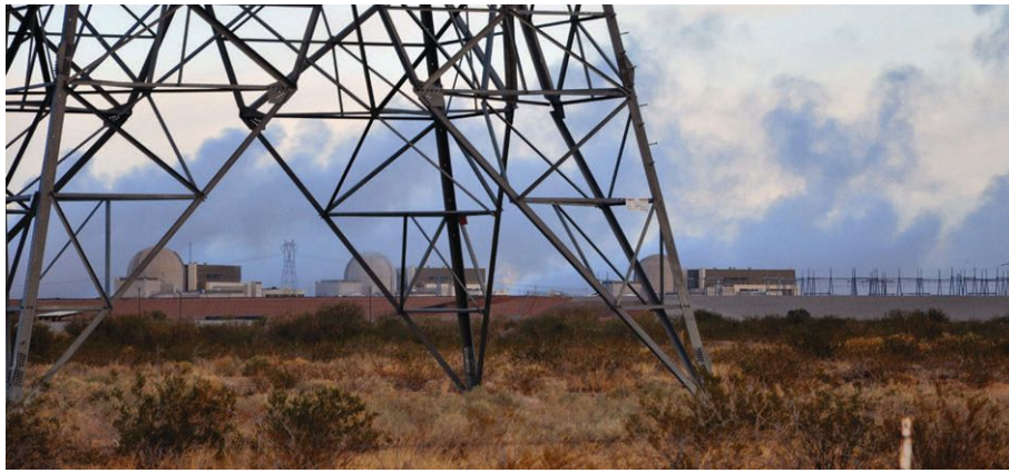
Figure 4 | Palo Verde's mission is to safely and efficiently generate electricity for the long term. The three units generate enough electricity for more than four million customers in the Southwest U.S. Palo Verde area, and directly and indirectly supports an estimated 8,800 jobs and has an annual economic impact on the Arizona economy of $1.8 billion. (Photo courtesy of Palo Verde Nuclear Generating Station.)
