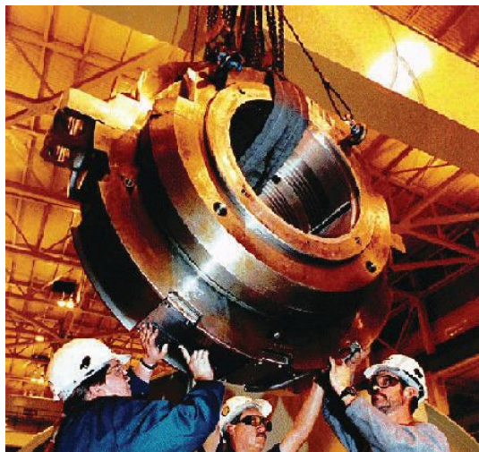
Figure 2 | A bearing being removed from a turbine. The bearing supports the shaft. There are two bearings for each high and low pressure turbine unit. The bearing vibration and temperature are monitored continuously during plant operation. (Photo courtesy of Nuclear News.)
