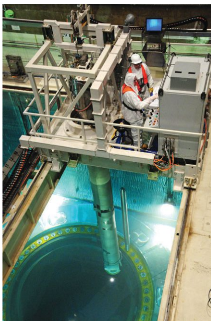
Figure 3 | Palo Verde refuel personnel coordinate a recent core reload in the unit Control Room and Fuel Building. Each of Palo Verde’s three units has approximately one-third of its 241 fuel assemblies replaced with new assemblies during refueling outages that take place about every five years in each unit. (Photo courtesy of Palo Verde Nuclear Generating Station.)
