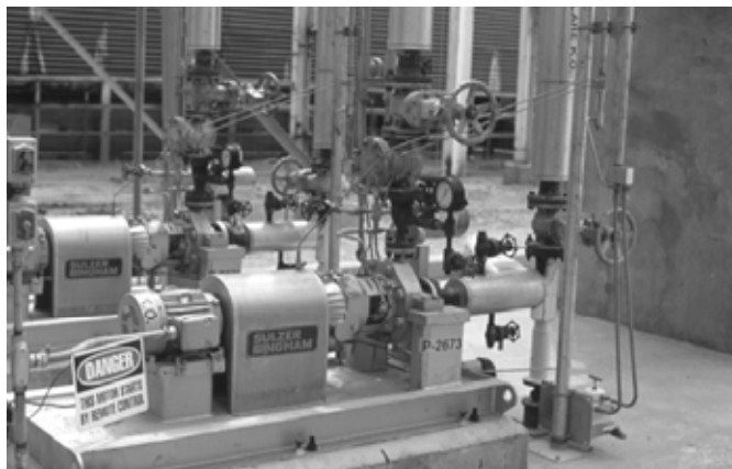
Figure 4 | Pure Mist Pump [Courtesy of Heinz P. Bloch, P.E. — Process Machinery Consulting]
